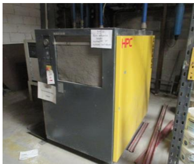
Keaser TE91 compressed air dryer
