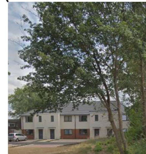
New housing - Franklins Court
